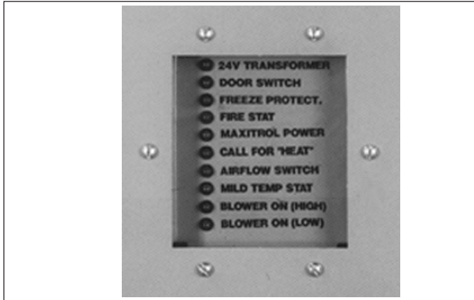
Figure 31.1 - Circuit Analyzer ①
